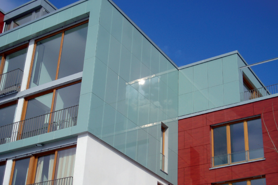
Apartment building, Dresden, glass façade fixed with FZP-G.
