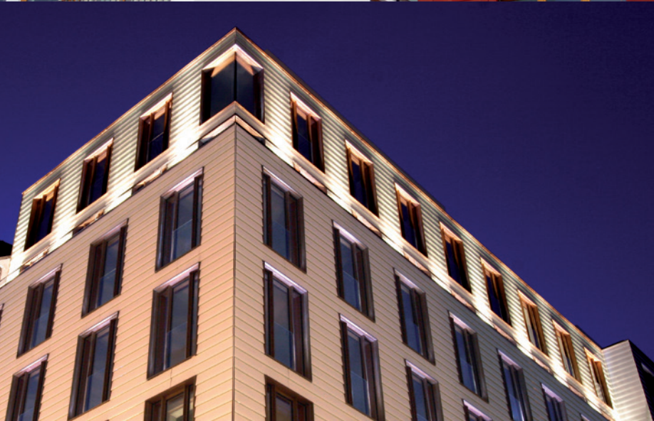
Neuer Wall 52, Hamburg. Glass shingle façade, fixed with FZP-G on SystemOne light.
