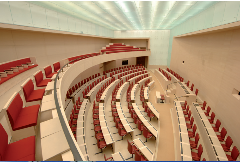
Assembly chamber, Bavarian Parliament, Munich, wall and overhead glazing fixed with FZP-G.
